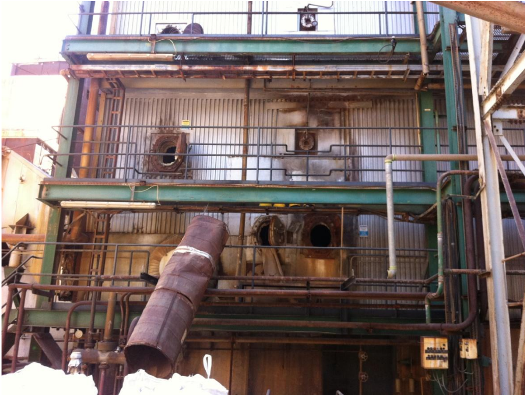
Figure 11. Boiler No 5. Entry Manholes
