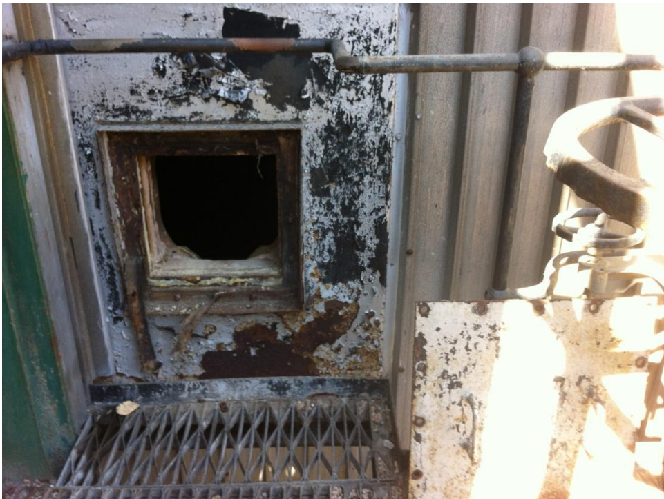
Figure 5.12 Boiler No 4. Entry to inner boiler through manhole on the LHS, north end of Boiler 4..
