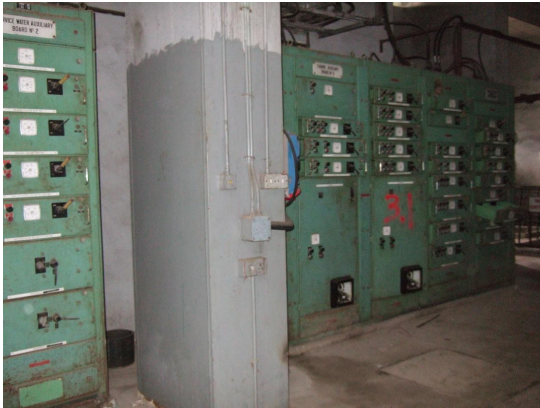
Figure 8. Location of various electrical switchgear along the east wall inside Turbine Hall containing ACM material
