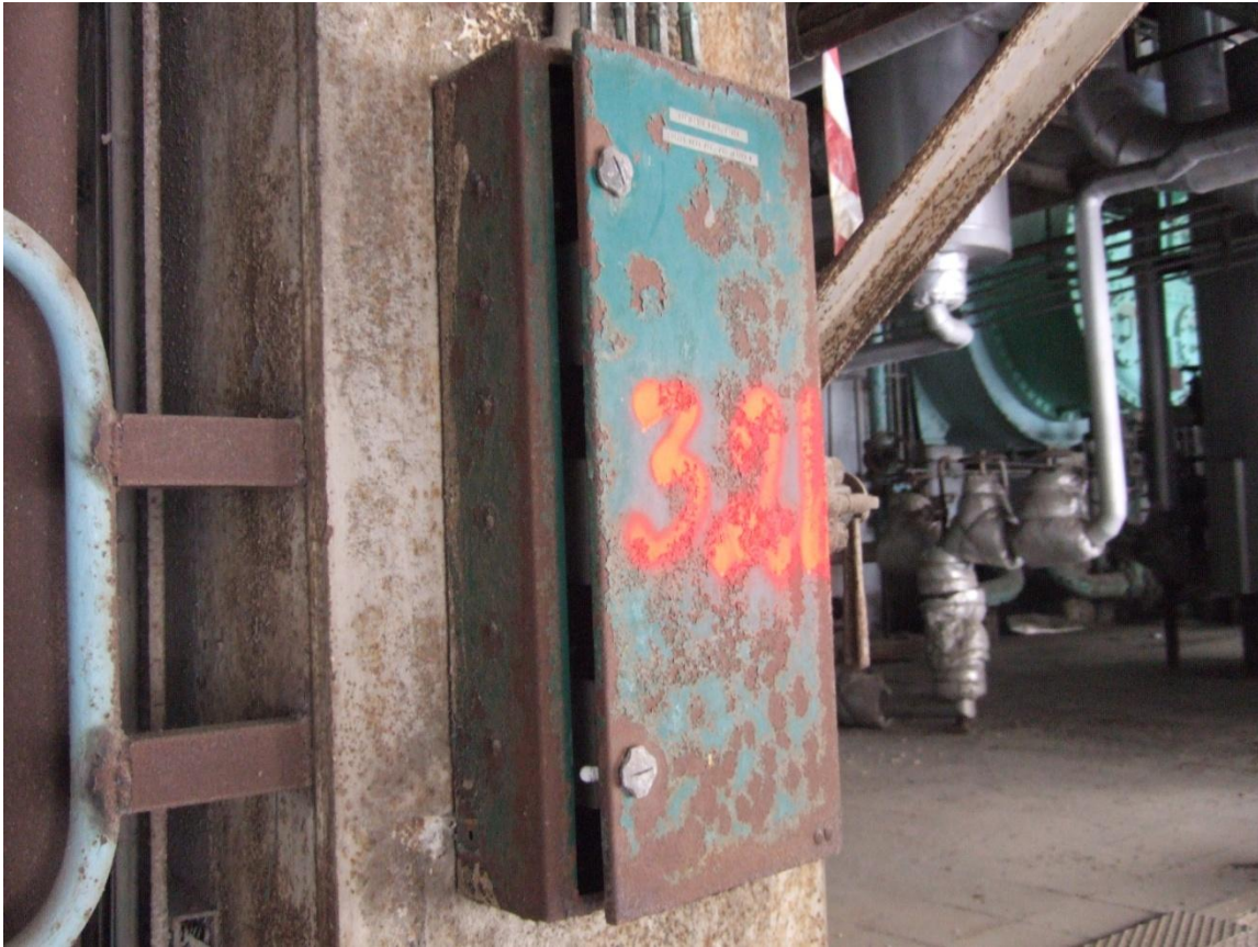
Figure 9 Typical Low Tension Switchgear with ACM on Ground Level ZONE 3.
