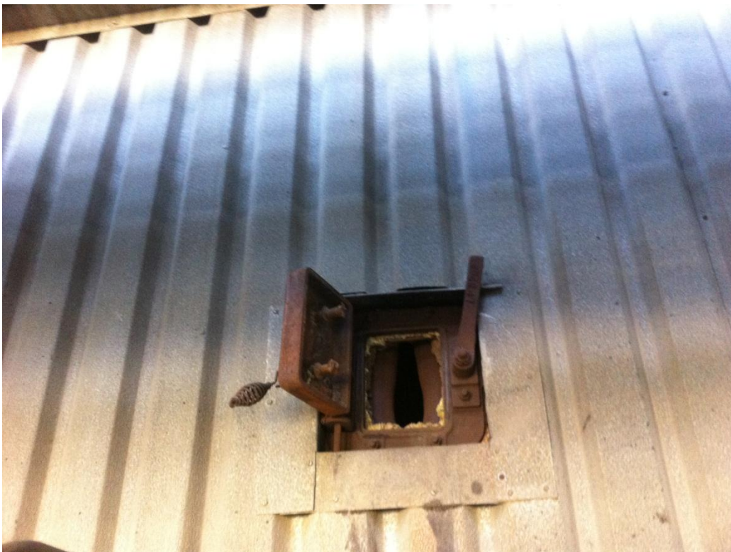
Figure 14. Boiler No 7 Open porthole, residue samples.
