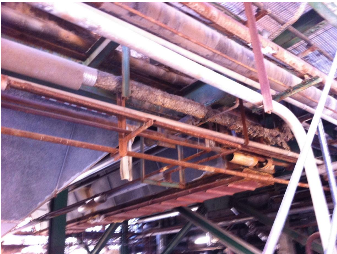
Figure 16. Boiler No 6. Sampling from exposed insulation tubing beneath Boiler.
