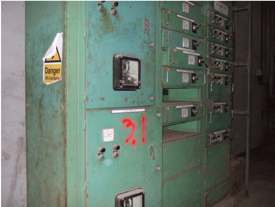
Figure 5. Location of various electrical switchgear along the east wall inside Turbine Hall containing ACM material
