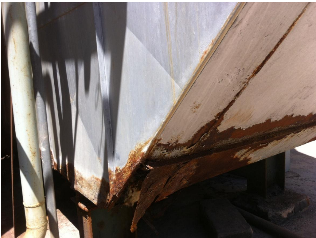
Figure 14. Boiler No 6. Sampling from exposed insulation.
