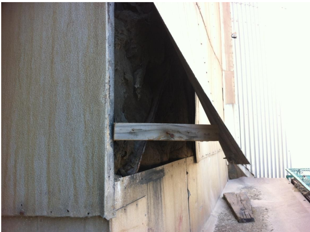
Figure 12. Boiler No 7 Insulation from underneath cover panels, north side.
