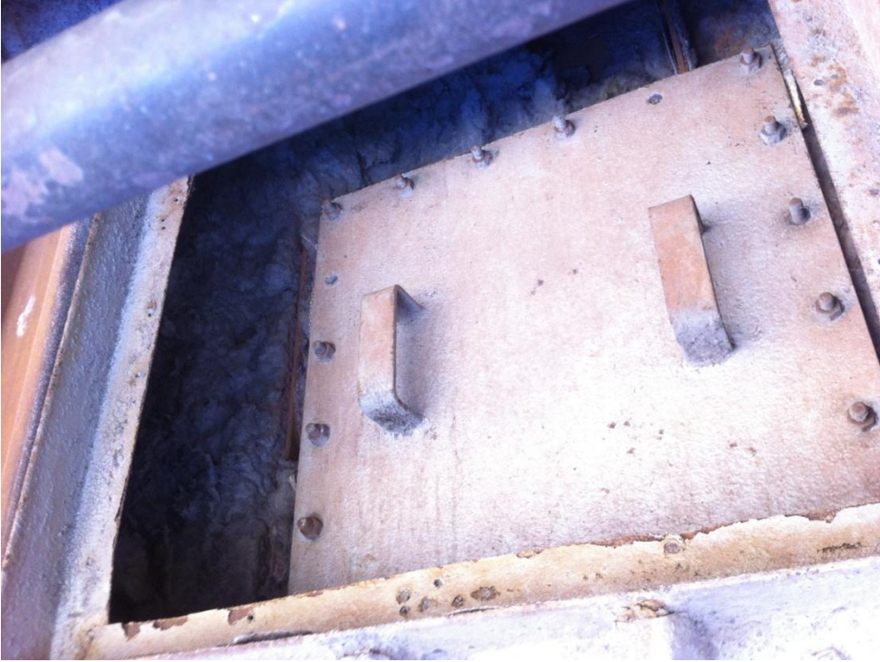
Figure 5.10 Boiler No 4. Sampling from side insulation over cover plate.
