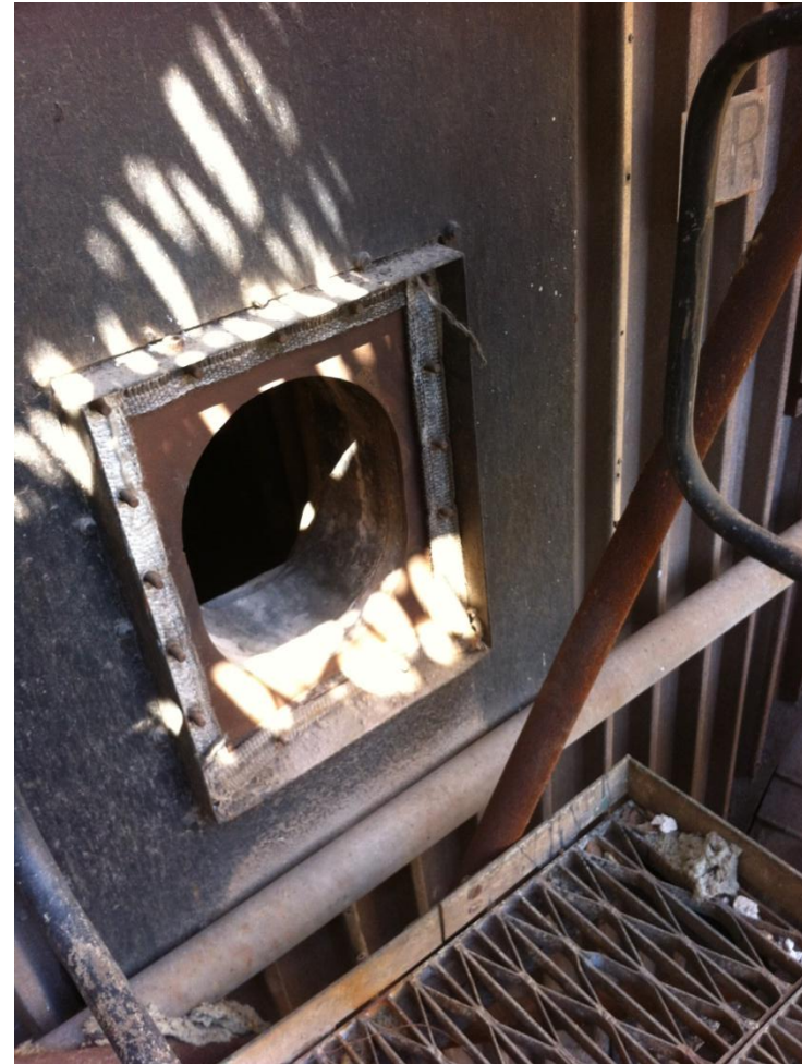
Figure 5.5 Boiler No 3. Entry to furnace through manhole on LHS of Boiler.
