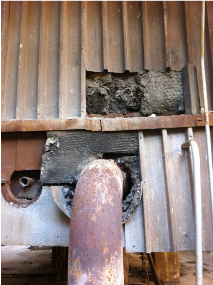
Figure 5.2 Boiler No 3. Sampling of insulation from opened side panel.
