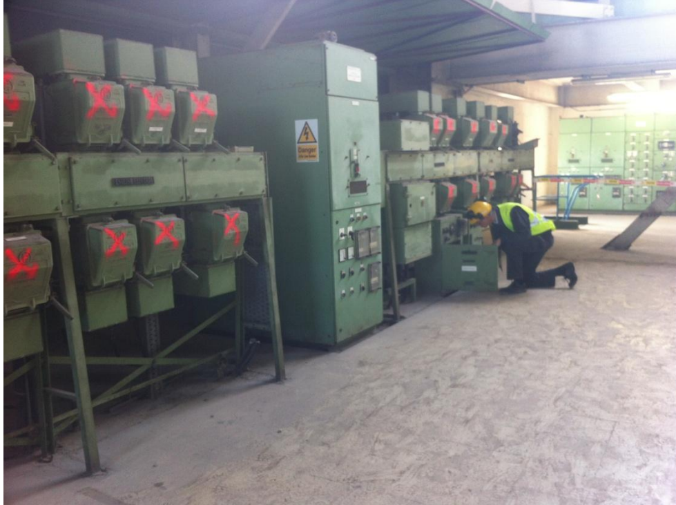
Figure 6 Location of various switchgear containing ACM material
