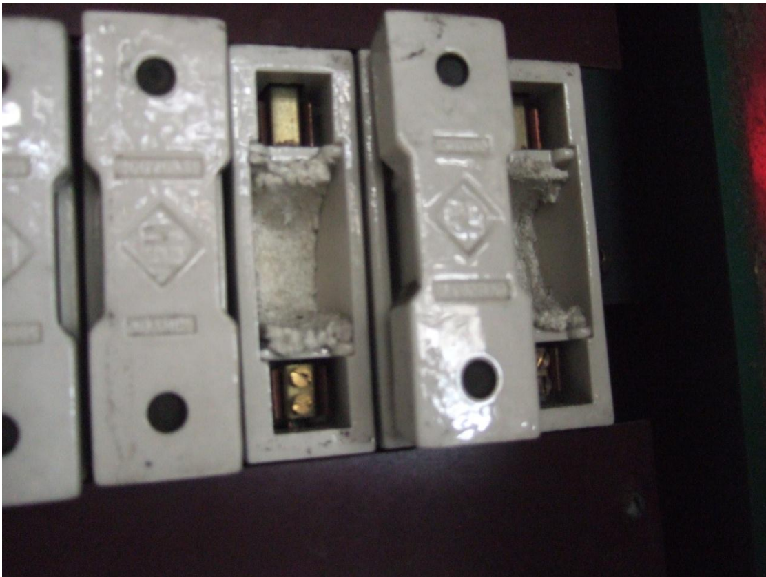
Figure 10 Typical ACM Liners present in Switchgear with ACM on three Levels ZONE 3.
