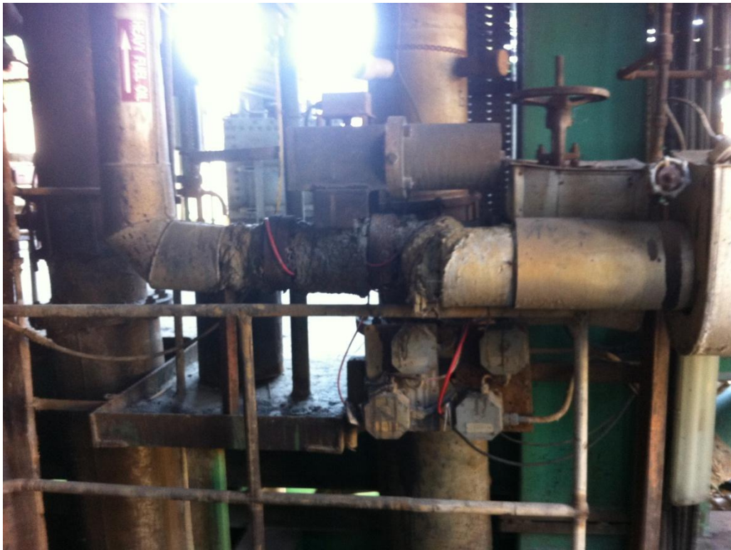
Figure 11. Boiler No 7 Various insulation from pipework
