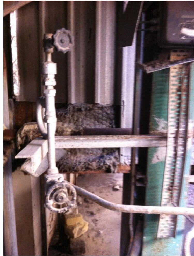
Figure 5.3 Boiler No 3. Sampling of insulation from opened side panel.
