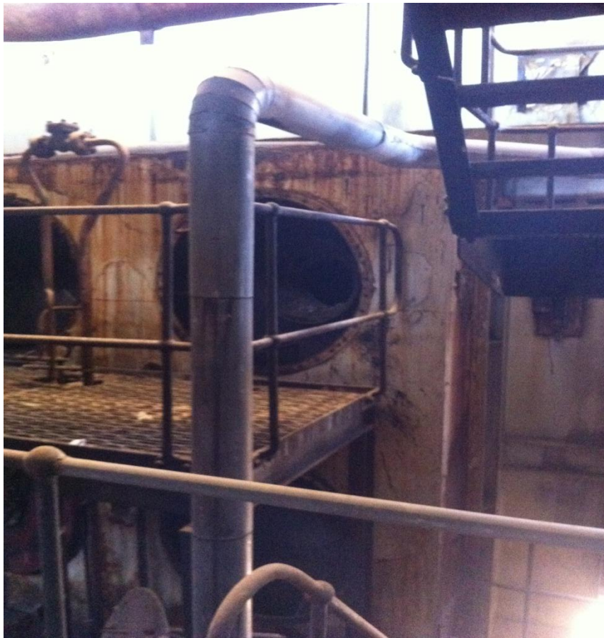
Figure 7 Presence of ACM Pipe Lagging in 2 nd Floor Level Boiler 2 ZONE 3.
