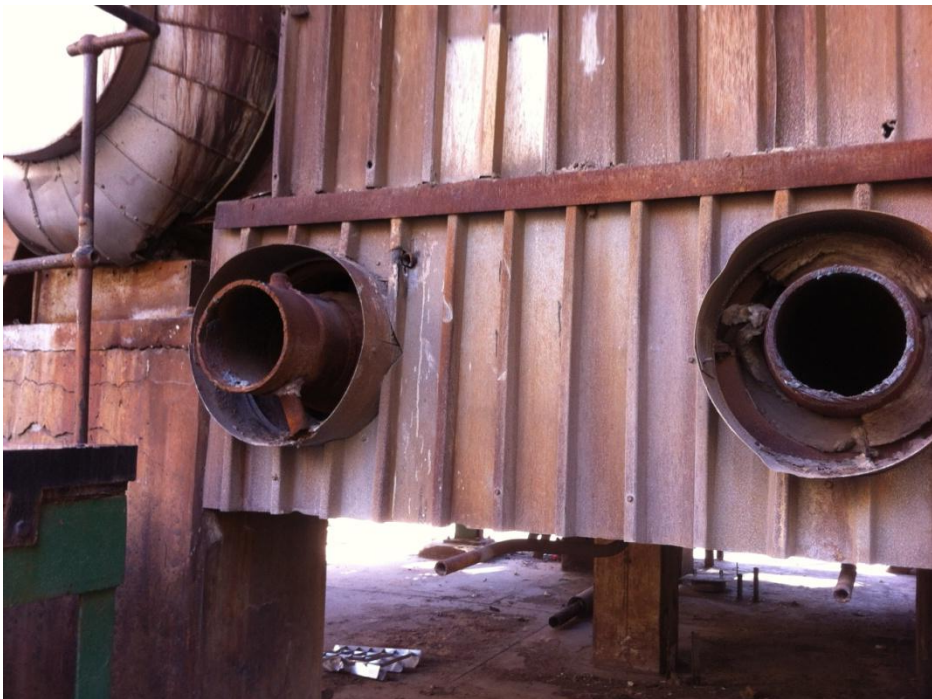
Figure 5.8 Boiler No 4. Sampling from side insulation over tubing.
