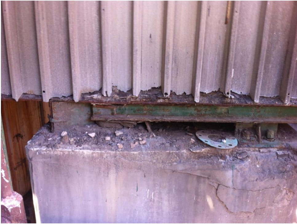
Figure 5.6 Boiler No 4. Sampling from behind rusted cover panels.
