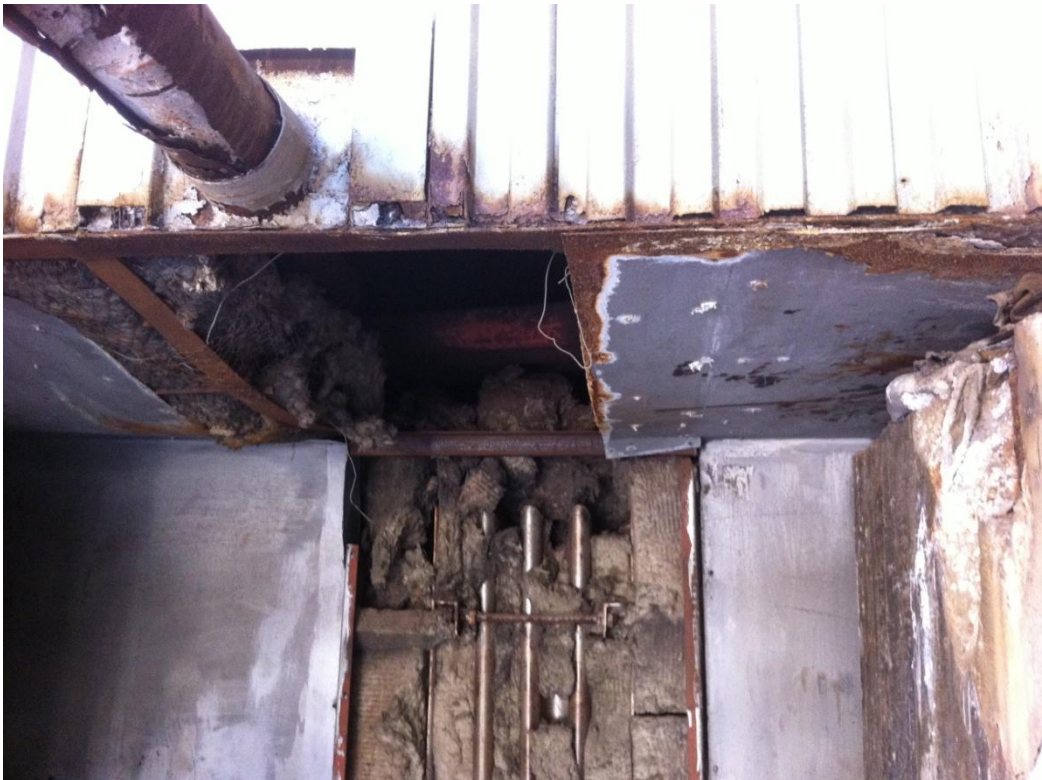
Figure 12. Boiler No 5. Access to insulation material through exposed outer panels
