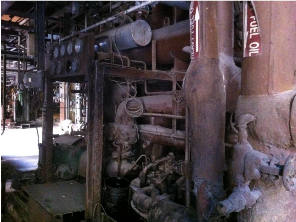
Figure 13. Boiler No 5. Various insulation materials covering pipework, in front of boiler.
