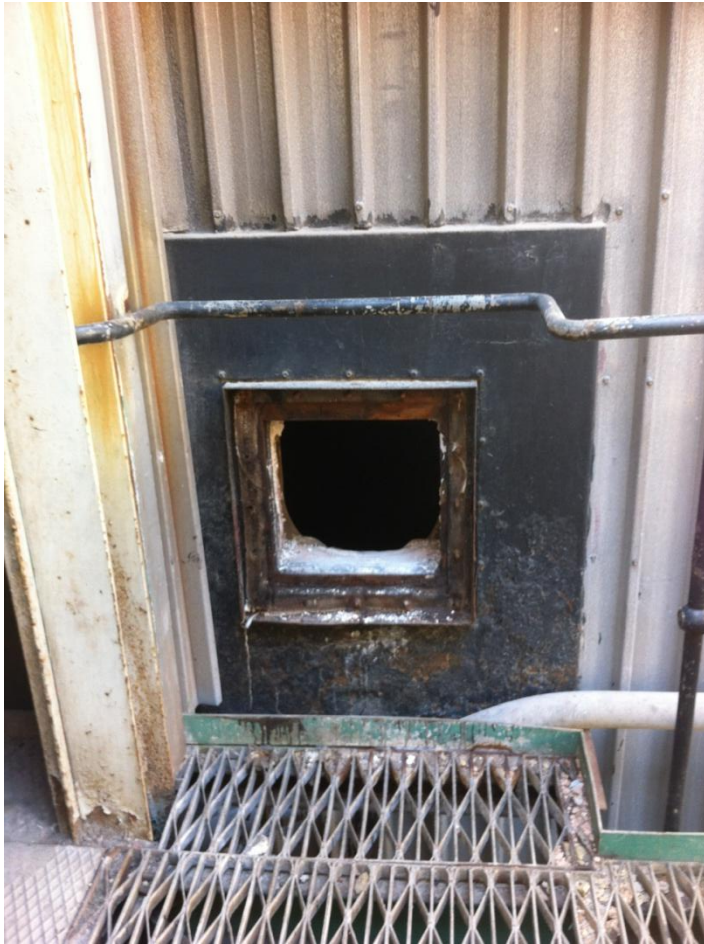
Figure 5.4 Boiler No 3. Entry to furnace through manhole on LHS of Boiler, north end
