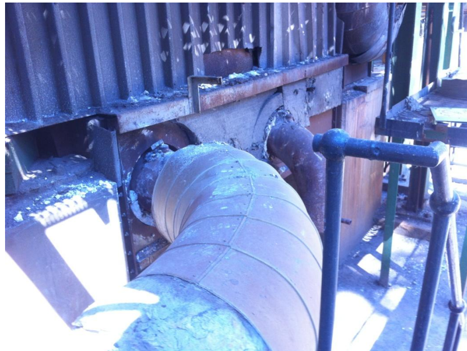
Figure 5.9 Boiler No 4. Sampling from side insulation over tubing.
