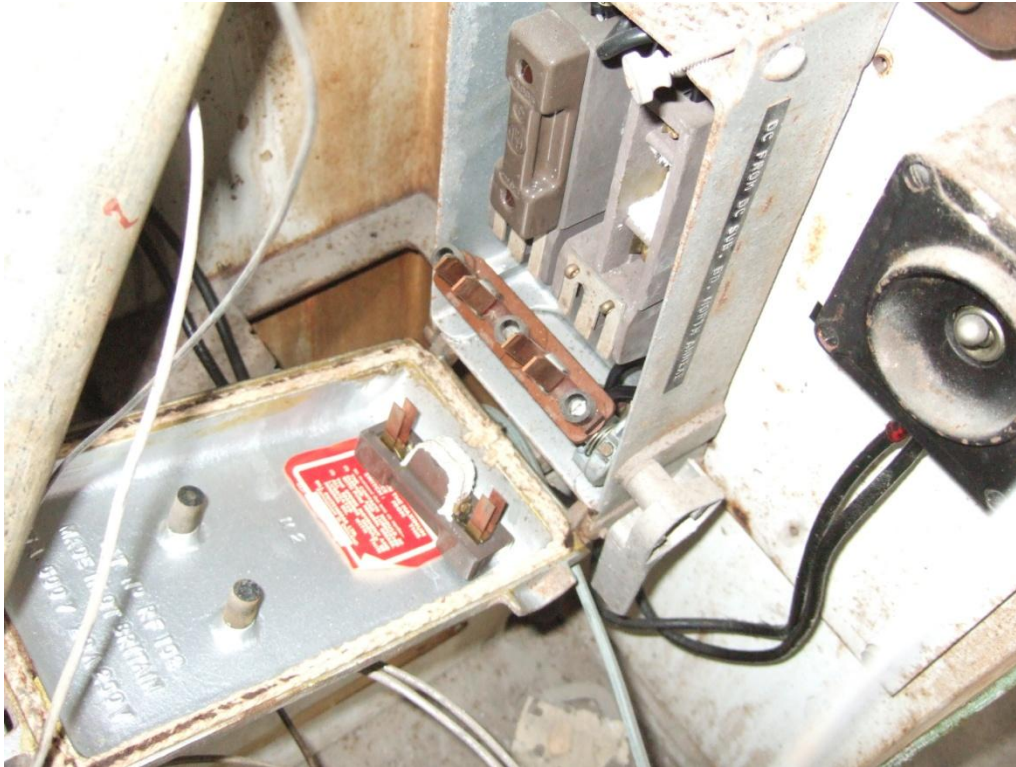
Figure 11 Typical, opened switchbox with ACM liners in ZONE 3.
