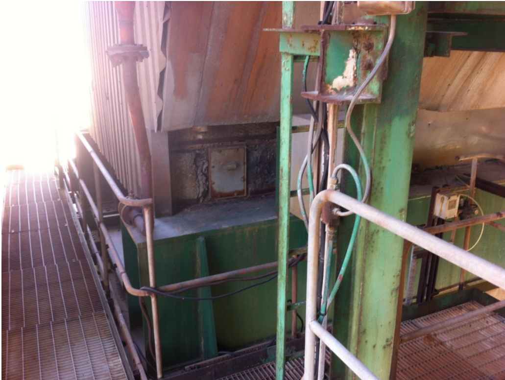
Figure 13. Boiler No 7 Insulation from exposed parts middle areas.
