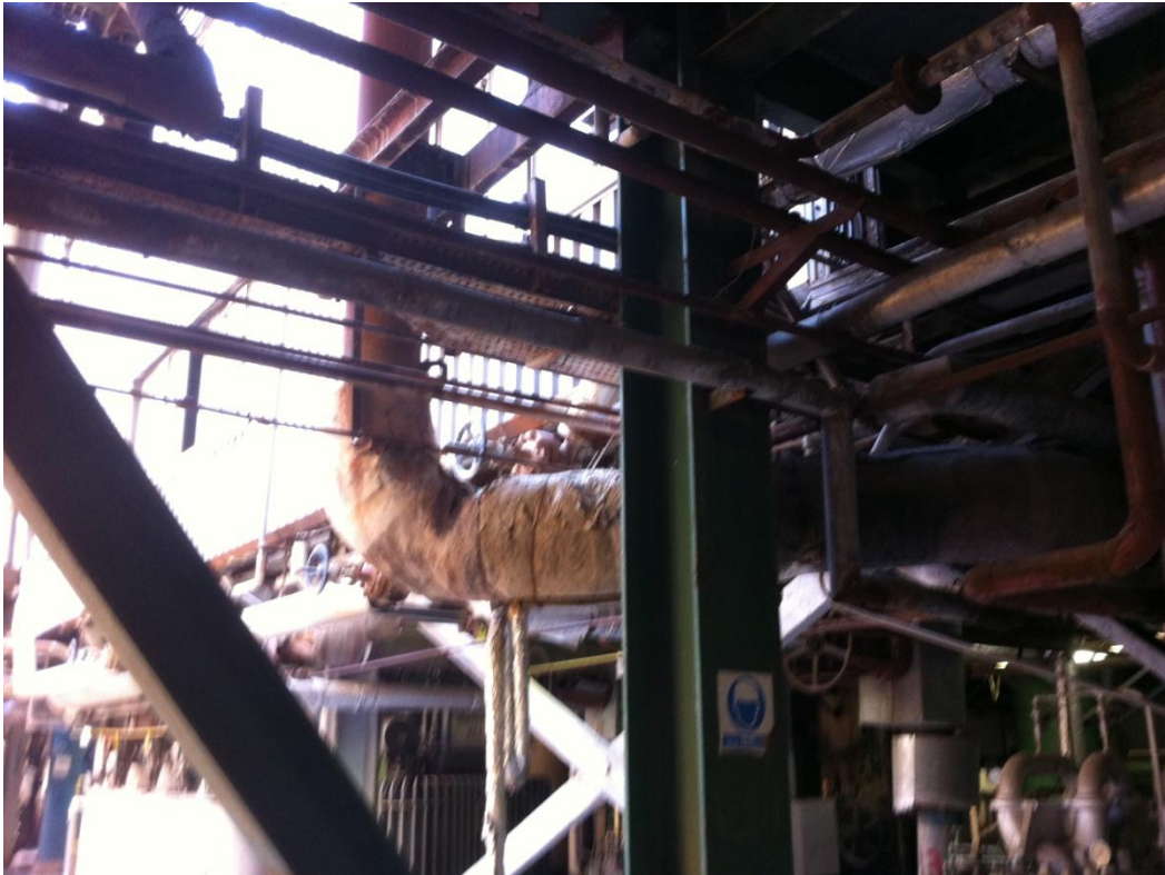
Figure 15. Boiler No 6. Sampling from exposed insulation covering tubing.
